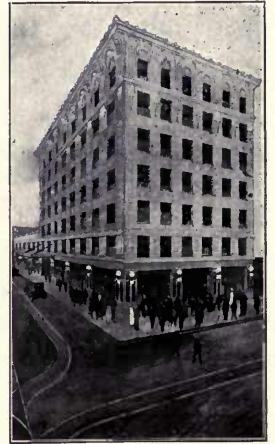
Illinois Traction System Bldg. now under construction.
